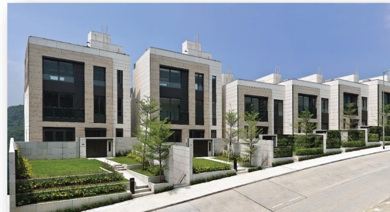
kau to HIGHLAND – Sha Tin
