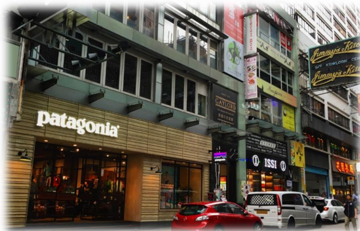
Nos. 21, 21A, 23-25 & 27 Ashley Road – Tsim Sha Tsui
